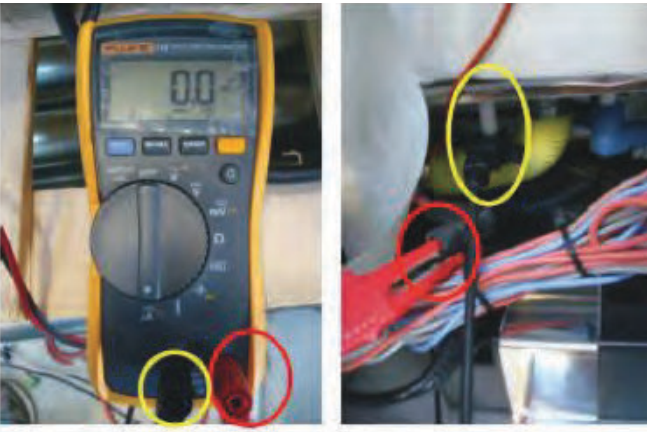
Figure 23 How to remove the flame detection cable
